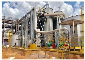
Clean TeQ Continuous Resin-In-Column Ion Exchange plant in DRC.
