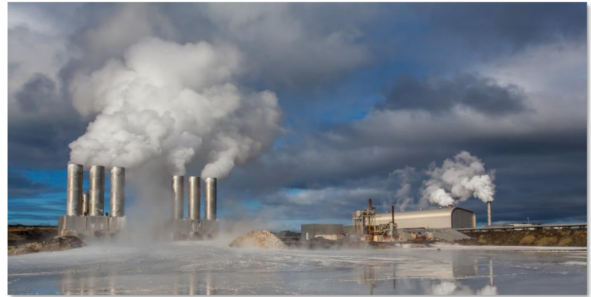
Geothermal Power Plant
